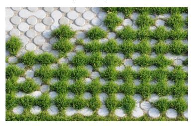
There are a wide range of 'grass block' concrete and polymer paving and ground reinforcing products that can enable the aesthetic and drainage benefits of a permeable grass verge to be retained, whilst also enabling its use for parking. An example is illustrated above. SAPC wishes to see consideration being given to the use of such products to enable the retention of the informal 90-degree parking layout, together with the aesthetic and drainage benefits of a permeable grass verge.
